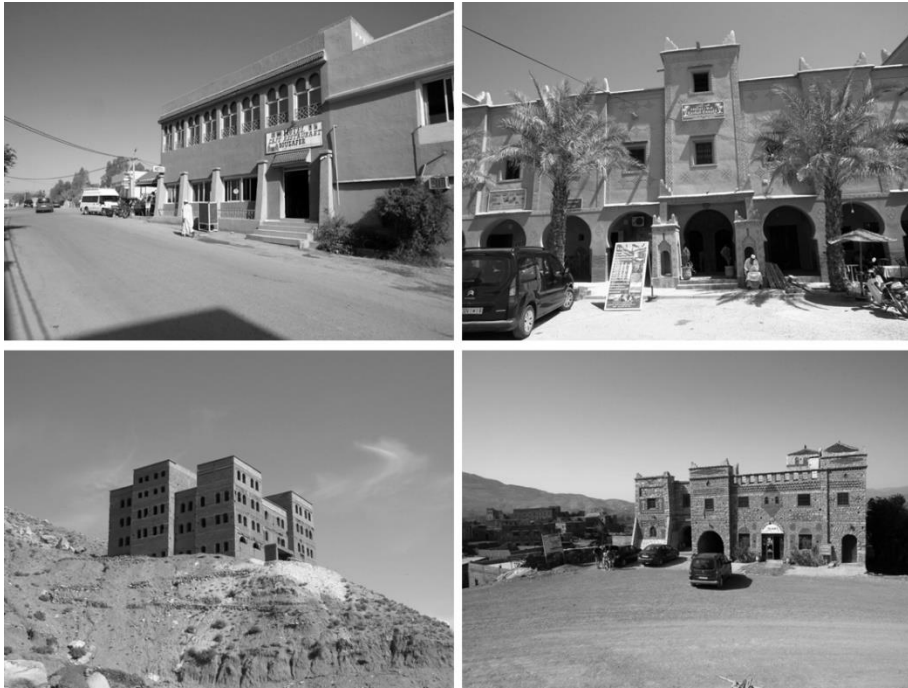
Figure 2: Newly built accommodation and restaurant facilities following the construction of asphalt roads (photos by the authors)
